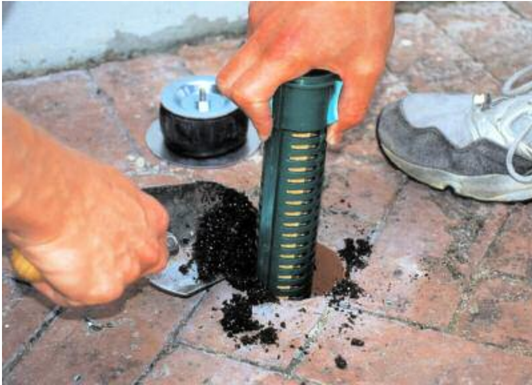
Figure D1.6 – Inserting a termite trap containing wood as bait
