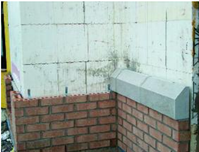
Figure 13.5 – Brick veneer construction on Amvic ICF
