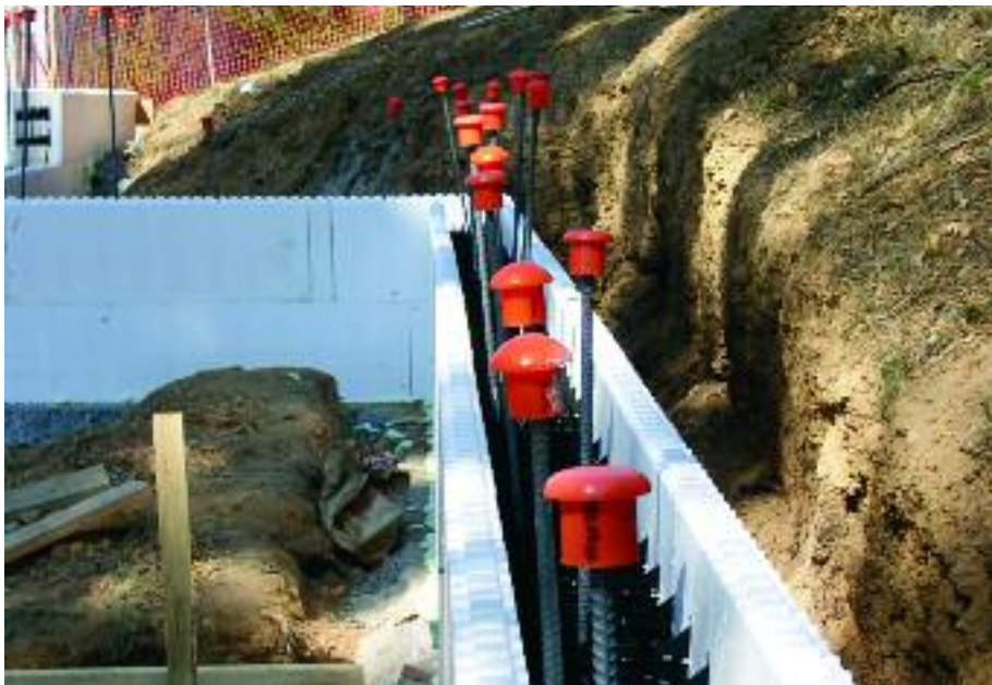
Figure 6.7 – Plastic mushroom caps on protruding steel bars
