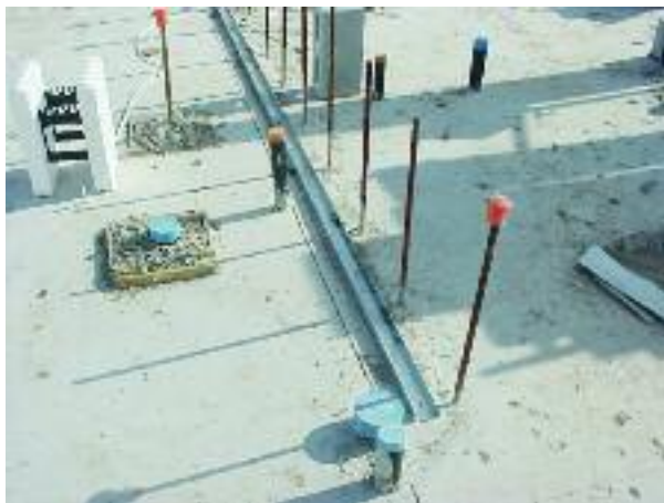
Figure 7.5 – Using a C-Channel to mark your wall layout
